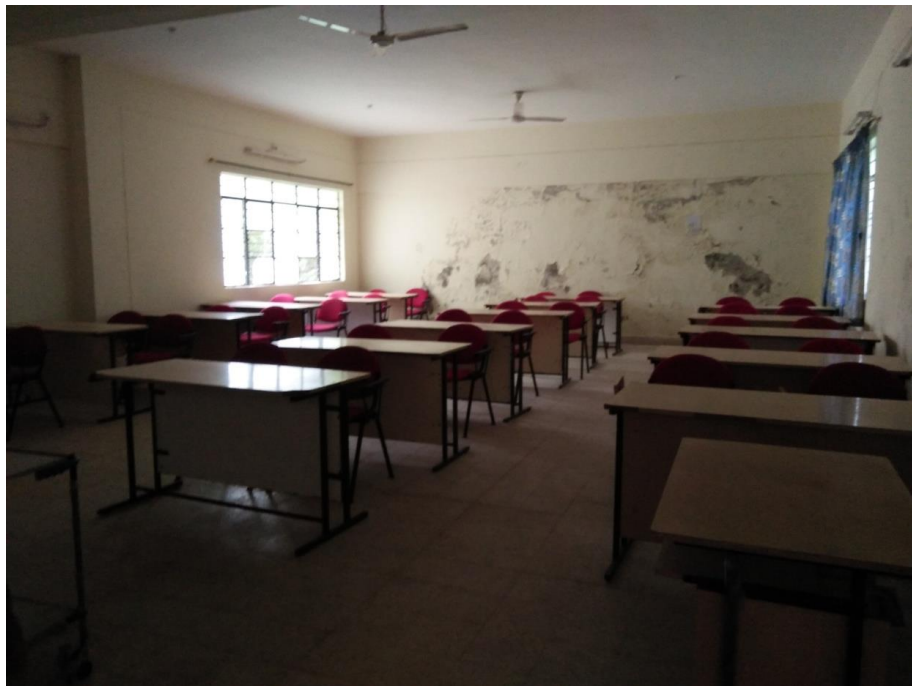
Figure 9: Training Centre in Raichuru
